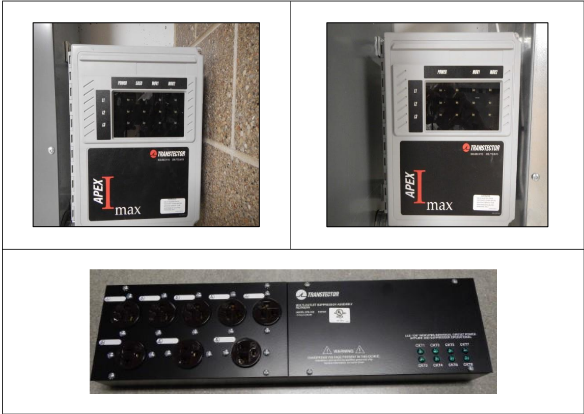
Figure 3e Surge Protection Device
