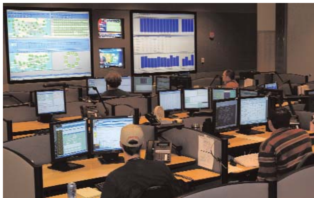
TCS' Seattle Service Bureau is the only TL-9000-certified facility providing wireless or VoIP 9-1-1 location services in the U.S.
