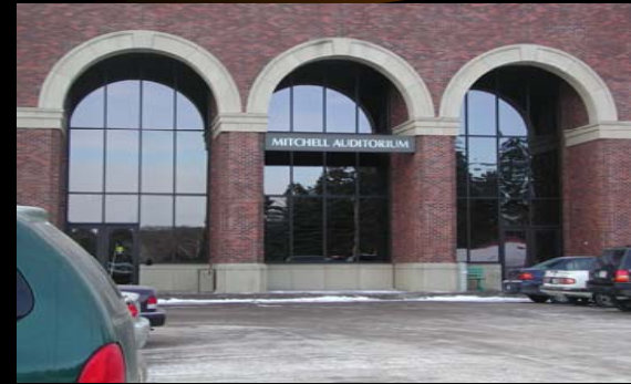
Mitchell Auditorium 1200 Kenwood Av.
